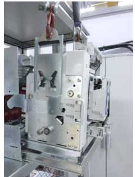
Placement of a draw-out DMX 3 in its base
