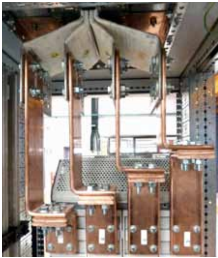
Kit for connection between a draw-out DMX 3 size 1 and an incoming SCP
