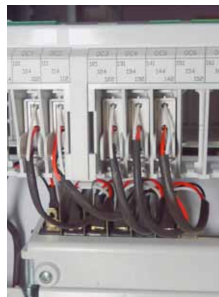
Four pre-installed auxiliary contacts and an optional auxiliary contact
