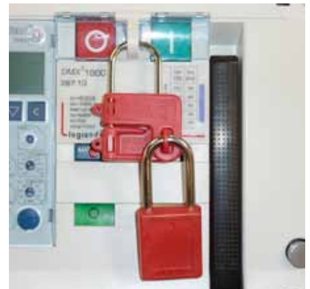
Padlocking the ON and OFF buttons
