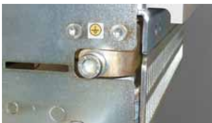
Connection point on the draw-out base
