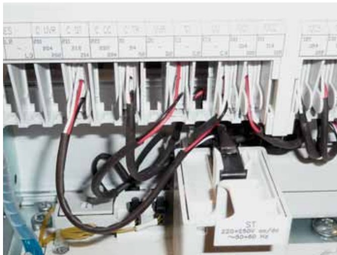
The signalling contact is mounted on top of the coil, trip unit or release
