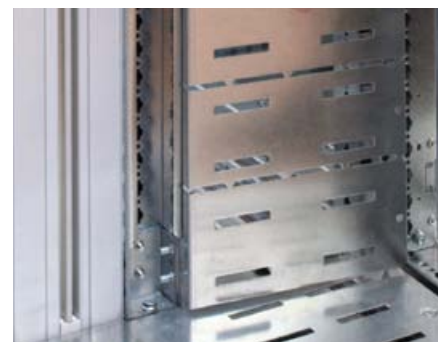
The spare compartments guarantee 3b form, required for IS 223, 233 and 333.
