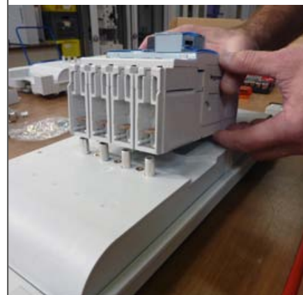
Place the circuit breaker on the movable part of the base.
