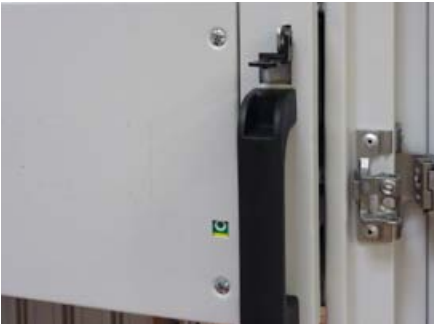
The tray position is indicated by a coloured LED and can be locked out with a padlock.
